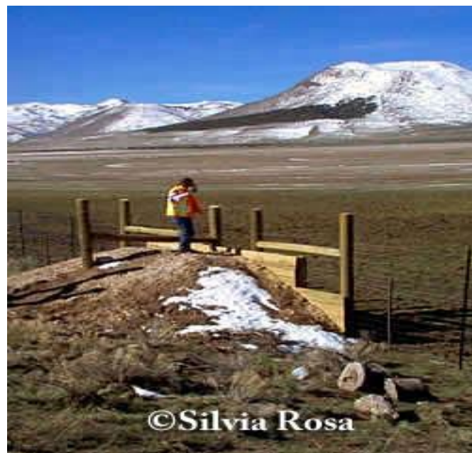
Figure 16: Escape ramp allows animals to exit but not enter
