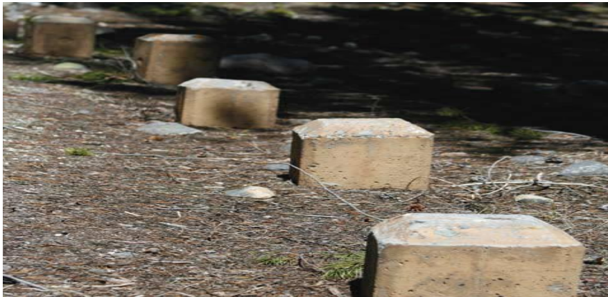
Figure 5: Large concrete blocks used to prevent vehicle entry
