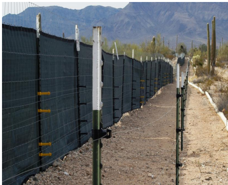
Figure 19: Hot-wire/ woven wire coyote enclosure with shade cloth for additional optical barrier Photo by AGFD / Jill Bright
