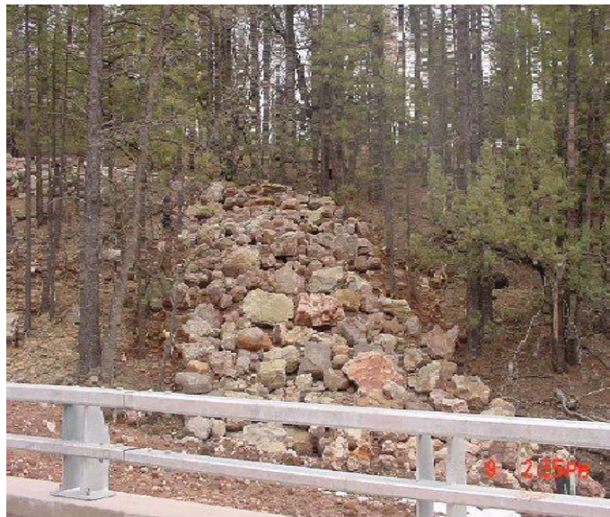
Figure 6: Rock "fence" used by ADOT to direct elk movements
