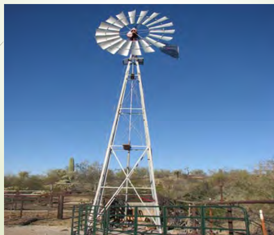
Pumping Plant - Windmill (533)
